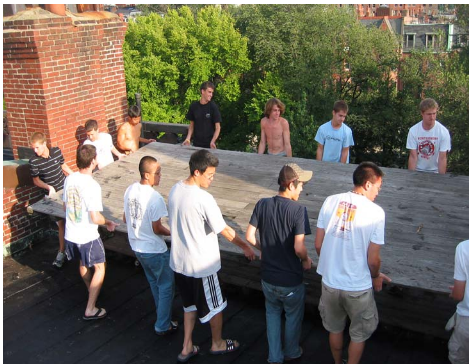
Brothers move the roof deck to prepare for retarring the roof. The roof leaks had been getting progressively worse, and the brothers retarred the roof as a short-term fix. Structural damage from water leaking is also becoming apparent.
